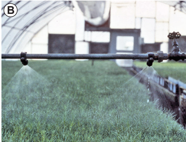
Figure 11.23 —Moveable boom irrigation systems (A) apply water in a very efficient linear pattern (B) but may be considered too expensive for many tropical nurseries. Photos by Thomas D. Landis.
