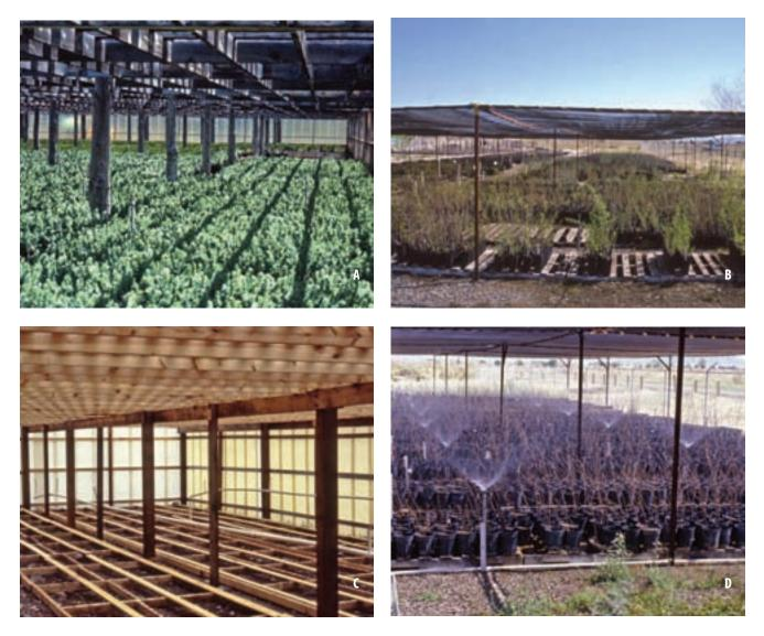
**Figure 4.8**—(*A*) Shadehouses are semicontrolled environments that are used for hardening and overwintering plants and (*B*) are also used for propagation. (*C*) They are constructed of wood frames with snow fencing or (*D*) metal frames with shadecloth and are equipped with irrigation systems that can also apply liquid fertilizer. Photos by Thomas D. Landis.
