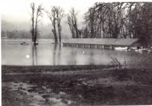
Figure 2.--Flooding of the equipment storage building ended operation of all nursery vehicles until they were reconditioned. Cedar shingletoe and peat moss were brought in by the current and heaped at the equipment shed as the waters receded.
