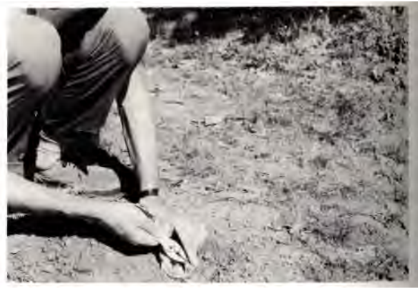
Figure 7.--Fill in the hole with topsoil: bend the tips of the lid back with pliers to make a 1-inch opening.
