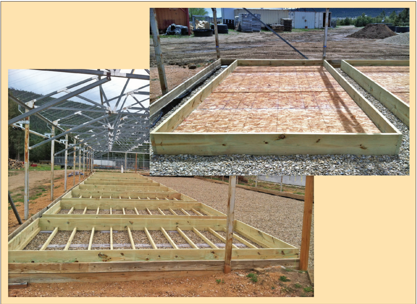
Figure 5. Subirrigation frame and flooring during installation process at the John T. Harrington Forestry Research Center in Mora, NM. (Photo by Tammy Parsons, 2015)
