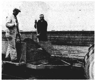
We have three wood frame sifters with different size mesh hardware cloth 1/4-inch for sand, 3/8 and 1/2-inch for sawdust. By adjusting the screen and the speed of the tractor to the material to be sifted the desired thickness of cover can easily be obtained.
