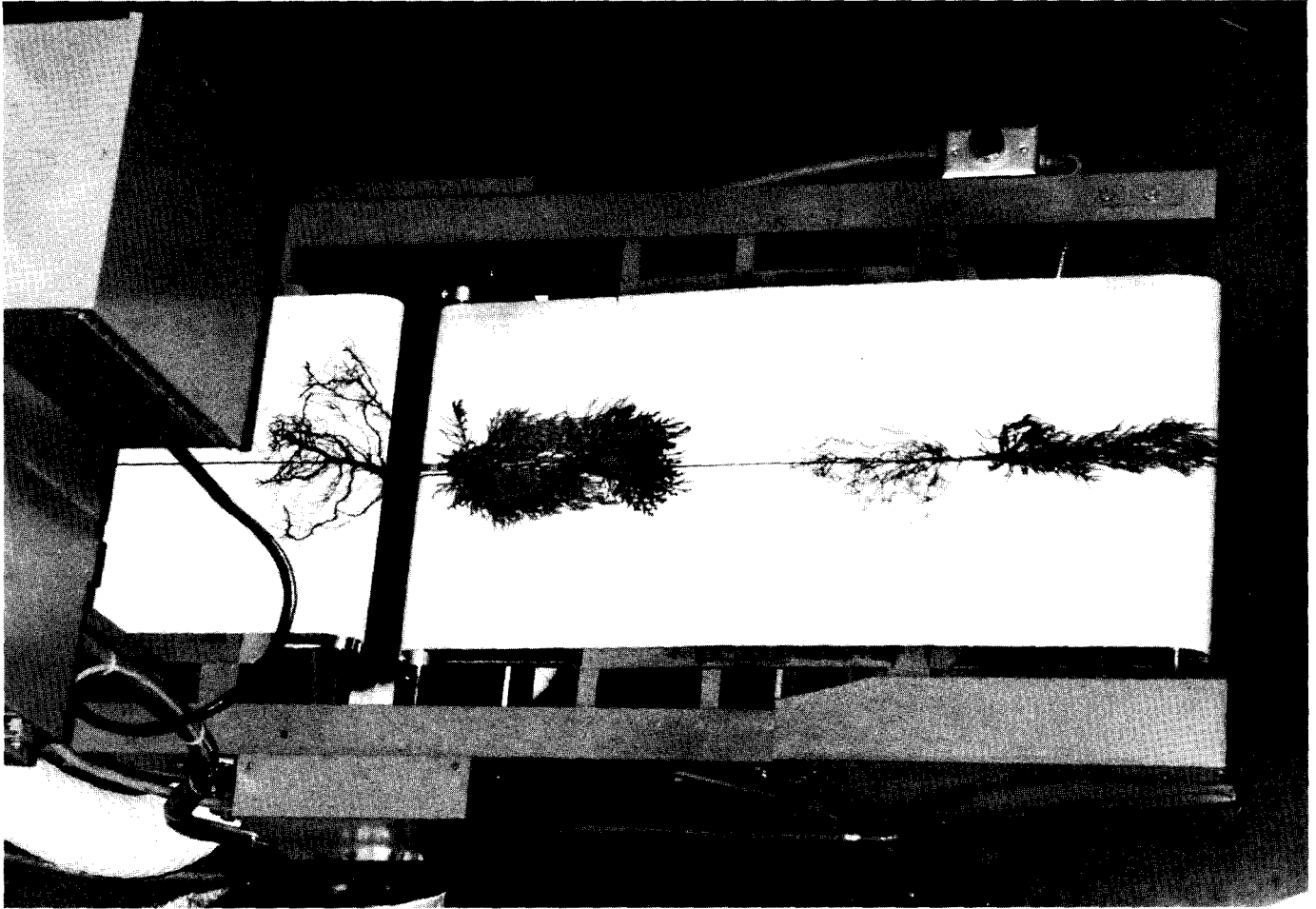
Figure 4—Machine vision quality control inspection station for tree seedlings.
