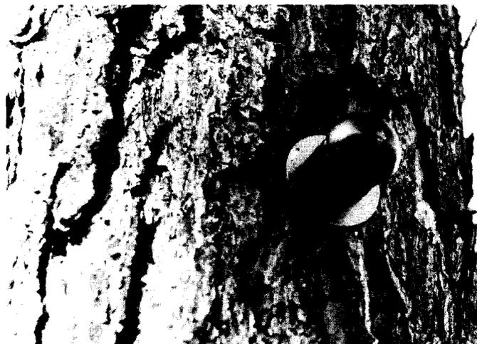
Figure 4—Lag screw installed in tree.
