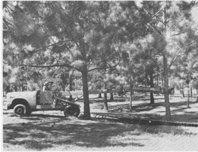
Figure 1.—Drive-over frame shown with shaker.
