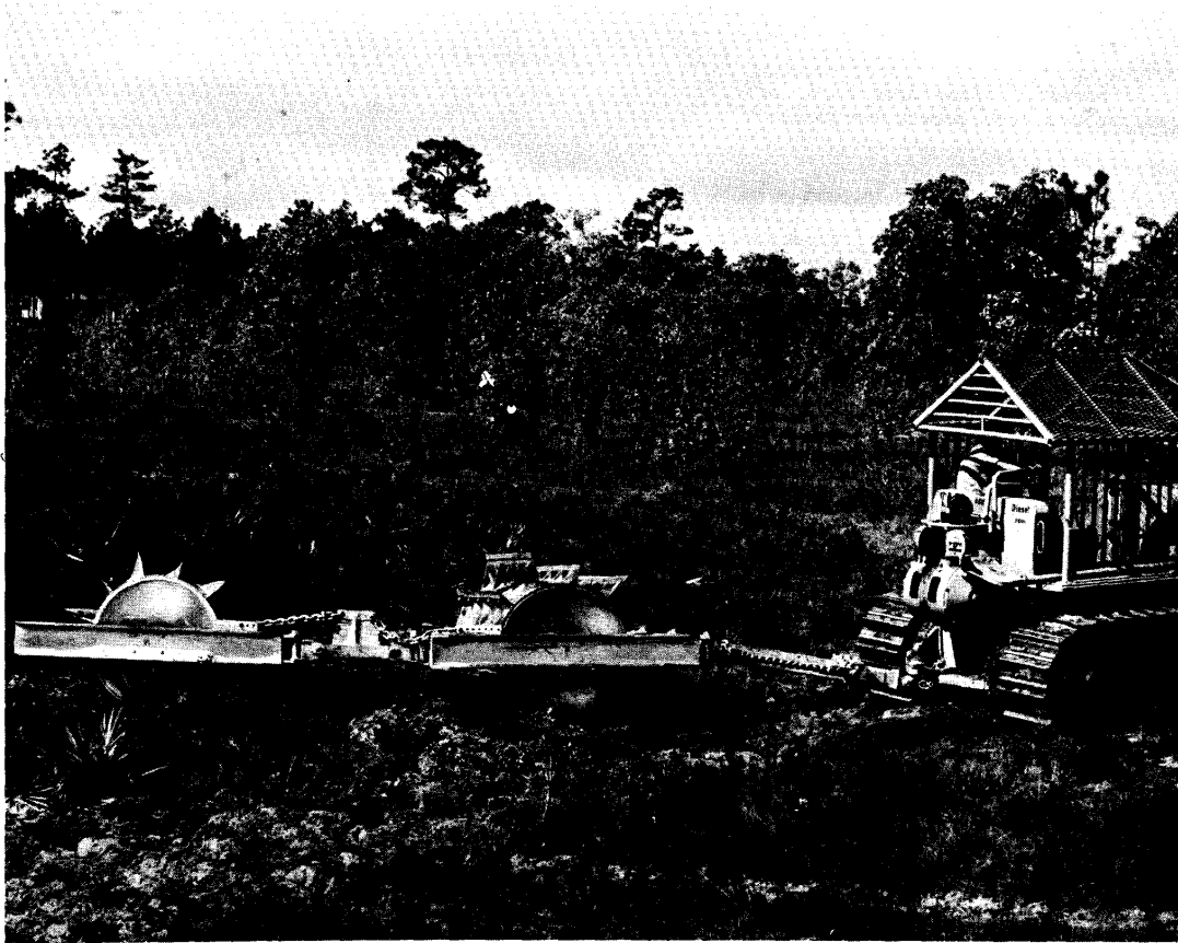
Figure 2.—Duplex chopper used in site preparation on the sandhills. During operation, both drums are filled with water.
