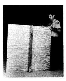
The 3 pieces of 2 inch x 4 inch x 4 foot framing and one of the 4 foot x 3 foot 103/4 inch plywood sheets are used as a platform or floor. One 2 x 4 is nailed to the cent& of the sheet of plywood parallel to the 4foot measurement. The other two 2 x 4's are nailed (one to each) to the bottom of the plywood sheets that are used as back and front walls (see photos 3 and 4).
