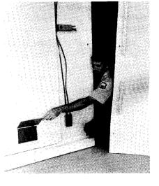
of .021 thick sheet metal, hinged at the top to allow air to flow through when the exhaust fan is activated, is placed over the opening.
