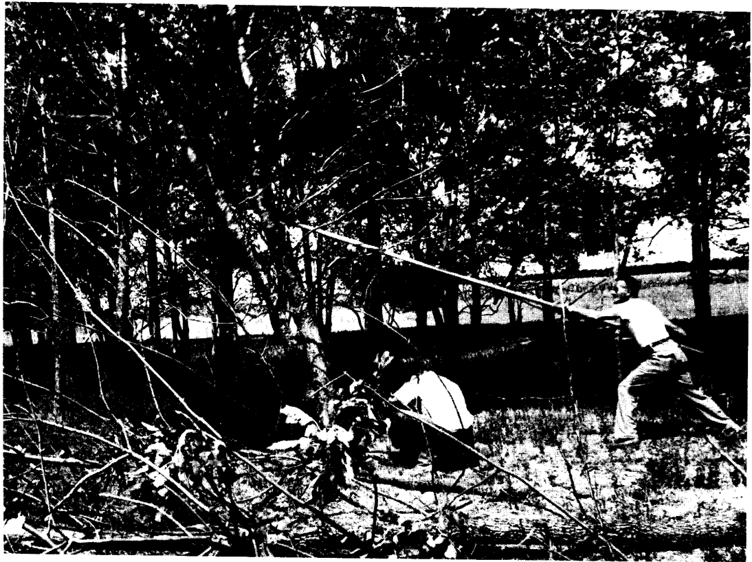
Figure 2.--Trees were cut at ground line with a chain saw and felled with a pike pole in windrows to make removal easier.
