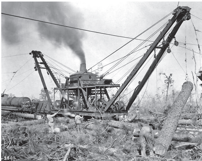
Figure 1. Steam-powered skidders manufactured by the Clyde Ironworks in Duluth, Minnesota, greatly increased logging capability in the early 1900s. Forty acres of timber could be skidded to the railroad track for loading on train cars with one setting of the skidder.
