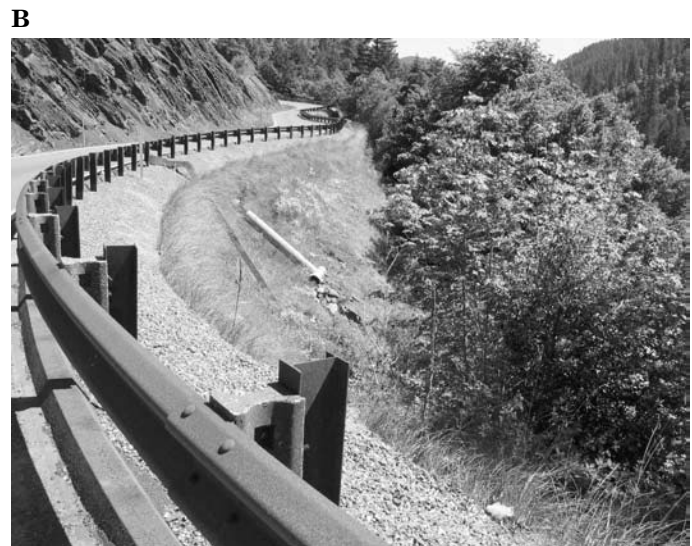
Figure 5 —In 2003, four months after gabion wall construction, seeded erosion mats were attached to the wire mesh at the face of the wall; compost amended soil was placed behind the screen and lightly tamped (A). Three years later (July 2006), the walls were fully vegetated and effectively screened from the road (B) (photos by David Steinfeld).
