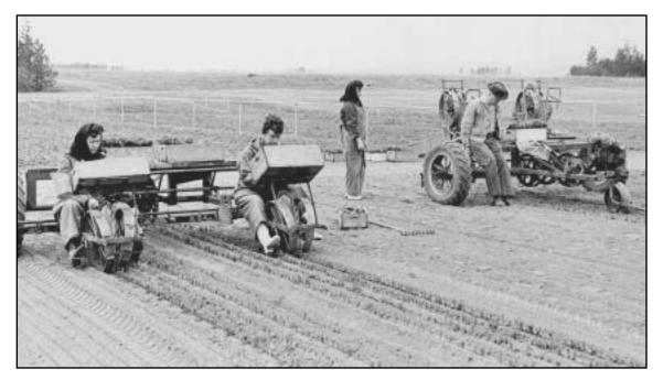
Figure 7. One of the first machine transplanters that was modified for tree nurseries was self-propelled and transplanted two rows at once.
