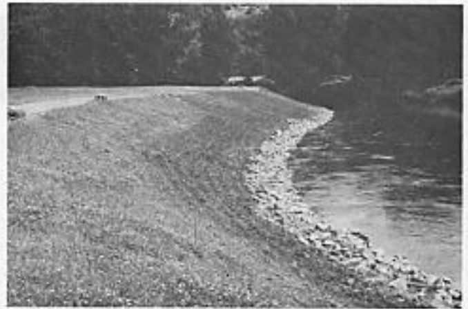
Figure 1.--Streambank planting along Green River, Washington; June, 1981, start of first growing season.
