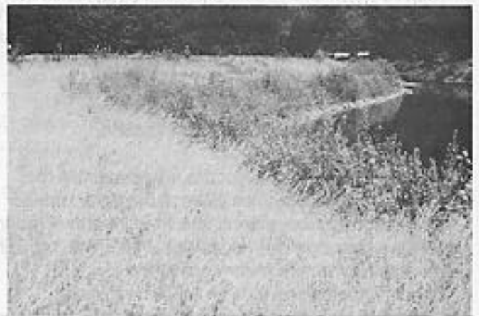
Figure 2.--By August 1983, shrubs perform well on lower bank; grass competition is severe on upper bank.
