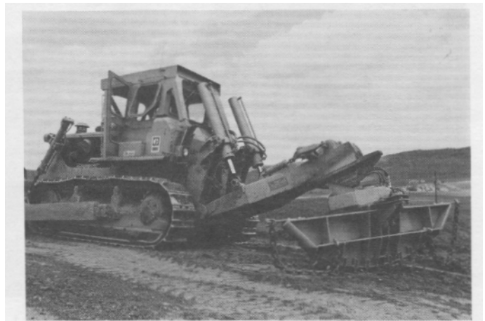
Figure 5.--Basin blade makes depressions in soil that trap moisture, creating favorable conditions for plant growth.
