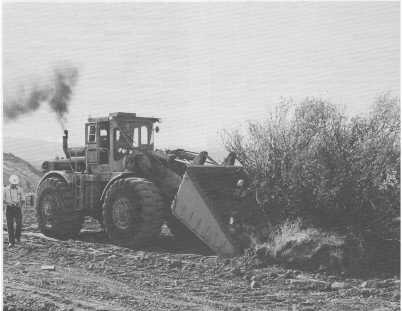
Figure 3.--Dryland sodder preserves topsoil and its vegetation for later replacement on reshaped spoil materials.
