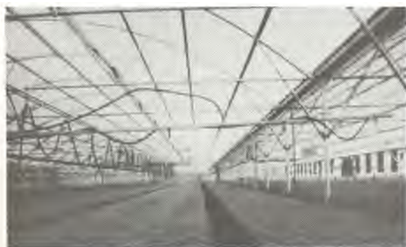
Figure 5.--Western hemlock seedlings growing in one section of the greenhouse. Hose loops of an irrigation system and a deflated heat distribution tube are visible at upper left.
