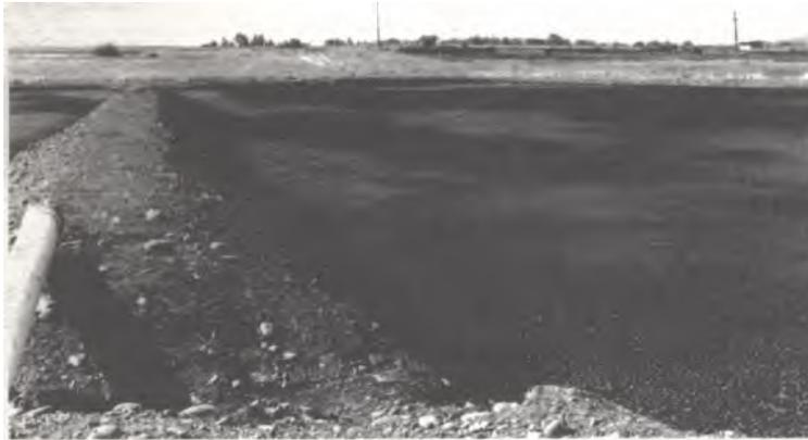
Figure 6. Sludge in drying beds following digestion. Vernon Thorpe Water Quality Control Plant, City of Medford.
