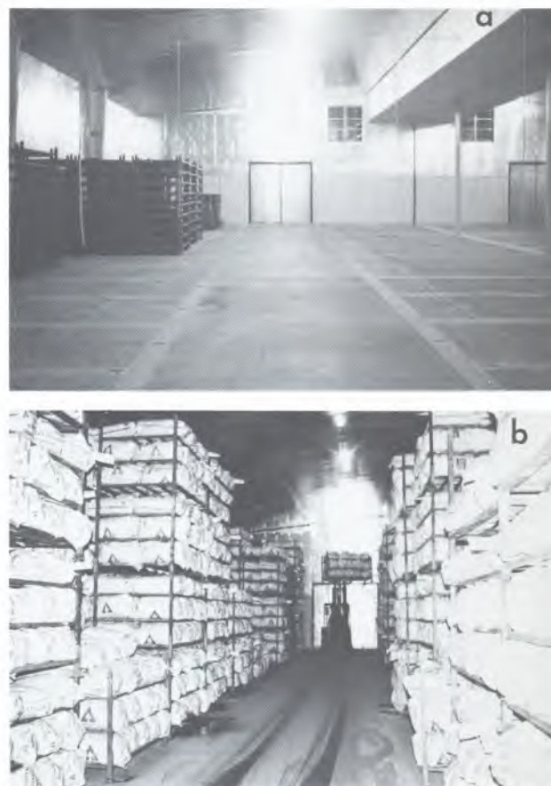
Figure 16.7. (a) Seedling storage cooler at Quail Ridge Nursery, Weyerhaeuser Co., Aiken, South Carolina. Note the rectangular structure at the middle of the ceiling. This is a plenum to distribute air in a circular pattern from the center of the room to the edge. The cords hanging from the ceiling at regular intervals are part of a network of thermocouples that monitor temperature. (b) Pallets of seedling bags are spaced to insure good air circulation.
