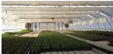
An energy/shade screen can be installed in a hoophouse. Tight sidewall seals are important.
