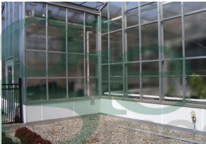
Thermax Heavy Duty Insulation as a kneewall on a gutter-connected greenhouse. Cost is about $1 per square foot.
