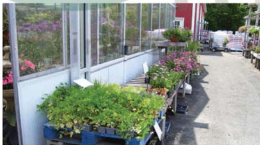
Thermax Heavy Duty Insulation as a kneewall on a gutter-connected greenhouse. Cost is about $1 per square foot.
