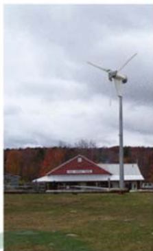
A 10-kw unit will generate 10,000-20,000 kwhr of electricity.
