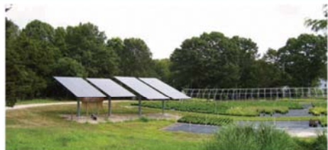
Solar requires good southern exposure for a minimum of six hours per day.
