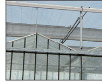
The main benefit to an exterior shade system is that light is intercepted before it enters the greenhouse.
