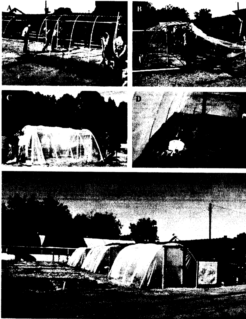
Fig. 2. Students in the Introduction to Horticulture (HORT 100G) class at New Mexico State University excavating a trench that will secure the plastic of a hoop house (A) and installing the plastic cover over a hoop house that has the door and frame completed (B and C); the interior of a completed hoop house showing a planted crop and data acquisition systems (D); three student-built hoop houses (E).
