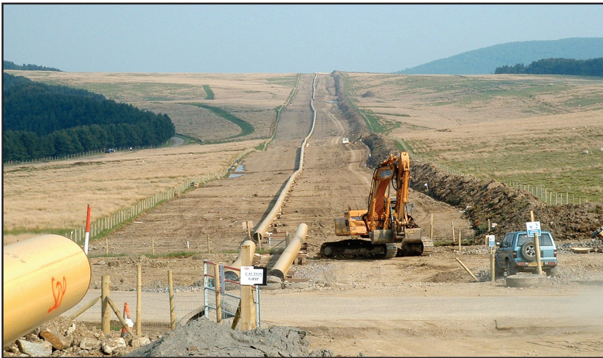
Figure 1. Brecon Beacons site during pipeline installation.
