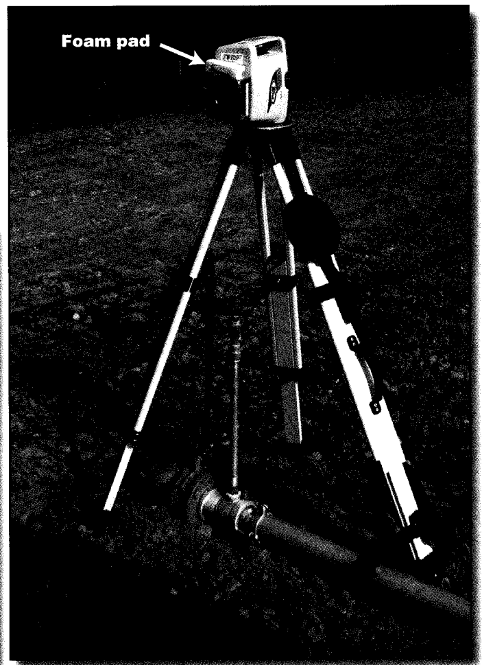
Figure 4—To help keep irrigation pipe in a straight line, the laser is centered and manually leveled over the irrigation pipeline's riser. The foam pad prevents the rotary laser's beam from being projected straight up where it could cause problems for aircraft pilots.
