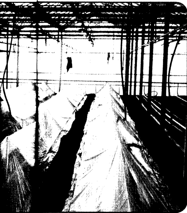
The sidewalls of this greenhouse were replaced with screen. Plastic can be rolled over the sides during cold weather.
