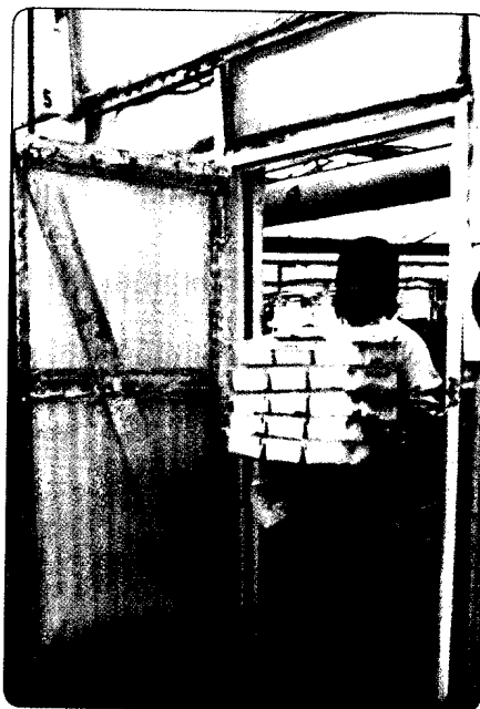
In greenhouses with a screened double-door entry, workers can prop the doors open to load crops onto trucks without allowing insects into greenhouses.
