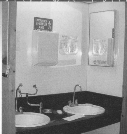
An eye-safety sink is accessible for workers at a greenhouse facility in Ohio.
