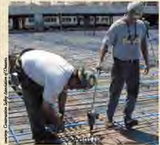
Manual rebar tying (left) vs. Use of an extended-handle rebar tying tool (right)
