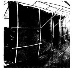
Engineering Services & Products Co. uses thermal mass in its greenhouses to store heat. The company developed black water bags to absorb heat and keep the greenhouse warm during the evening.
