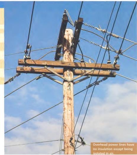
Step and touch potentials can occur when a tree trimmer or landscaper is working in an elevated position or on the ground near overhead lines. The location should be established such that the person and the longest conductive object he or she may contact cannot come within 10 feet for lines 50 kilovolts or less and more for higher voltages.
