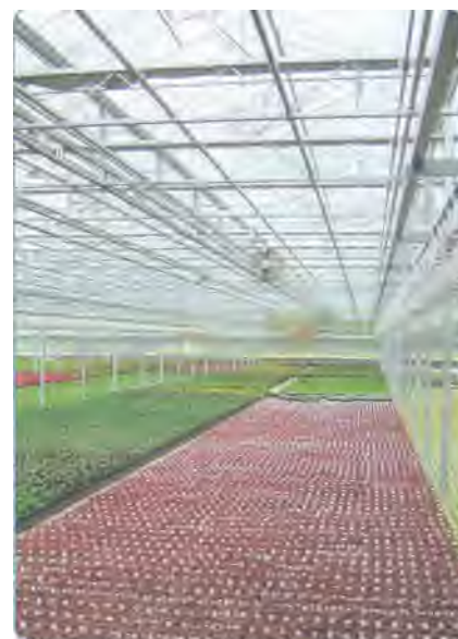
Floor heat is uniformly delivered directly to the root zone of a crop on the floor.
