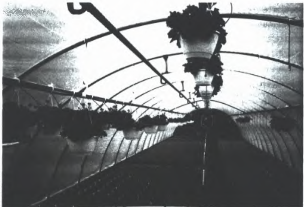
A tight greenhouse, while saving on energy, may result in high humidity, low carbon dioxide and high ethylene levels.
