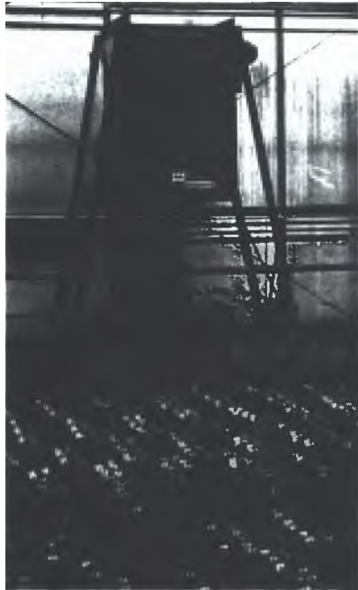
Tomato plants placed directly below this unit heater will indicate any ethylene given off by the heater.
