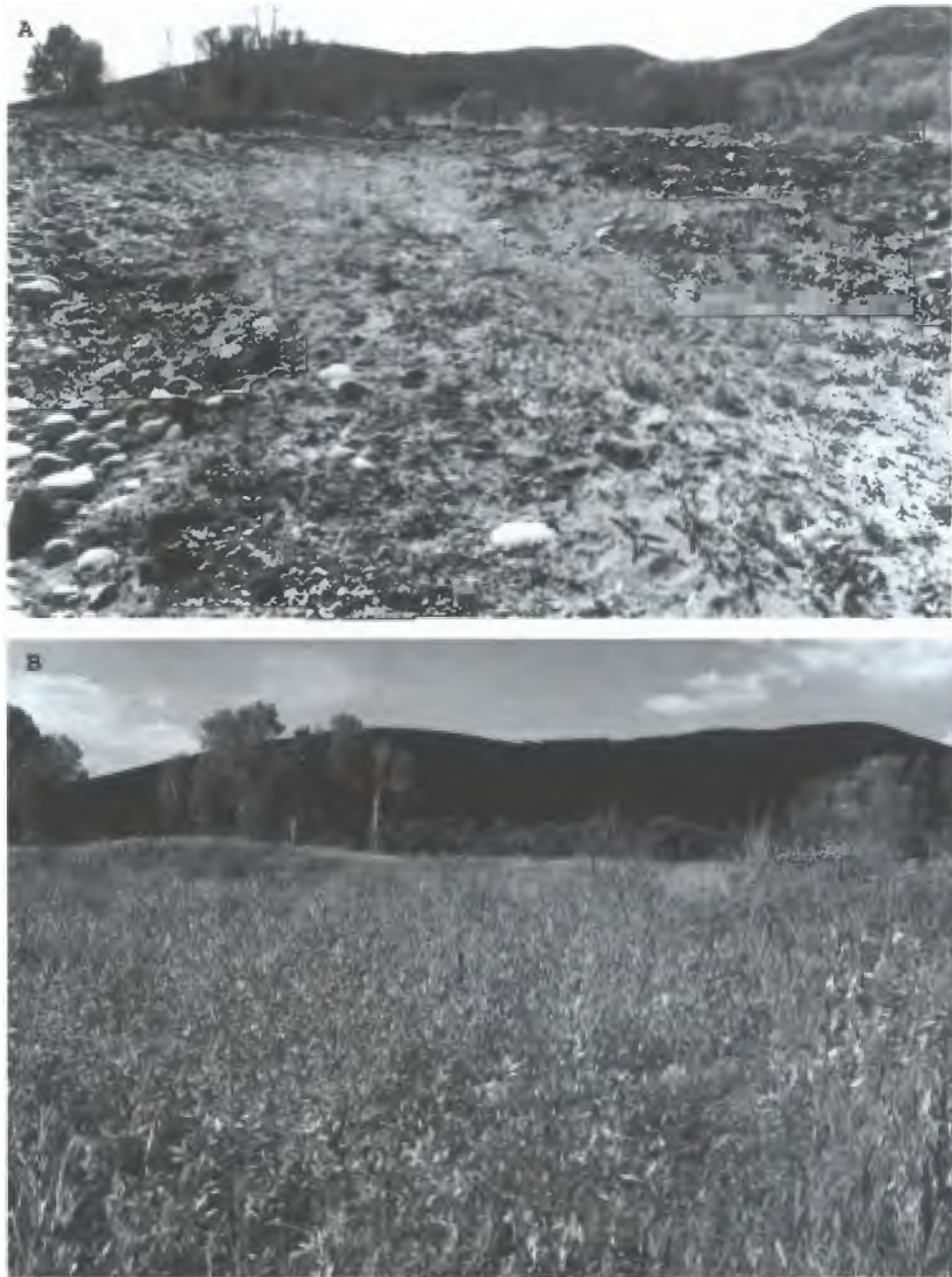
Figure 4—High flow channel one flood event after construction (A) and three flood events following construction (B). Note that no trees or shrubs have been installed at this location. Natural recruitment accounts for the many hundreds of seedlings.
