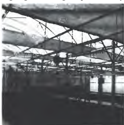
Internal energy/shade curtains can reduce energy consumption by 25-40 percent.
