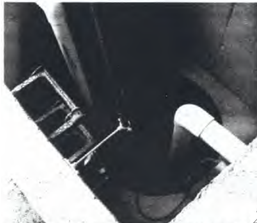
A common site in greenhouses is a ladder inside holding tanks. Growers routinely drain holding tanks several times a year and remove debris that collects at the bottom.
