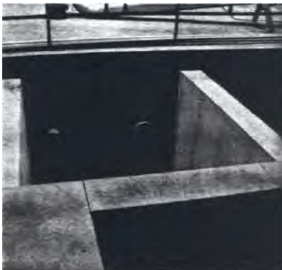
If concrete is not sealed, it can absorb water and serve as a habitat for algae, bacteria and fungi, which survive inside pores and resist conventional sanitizing treatments.
