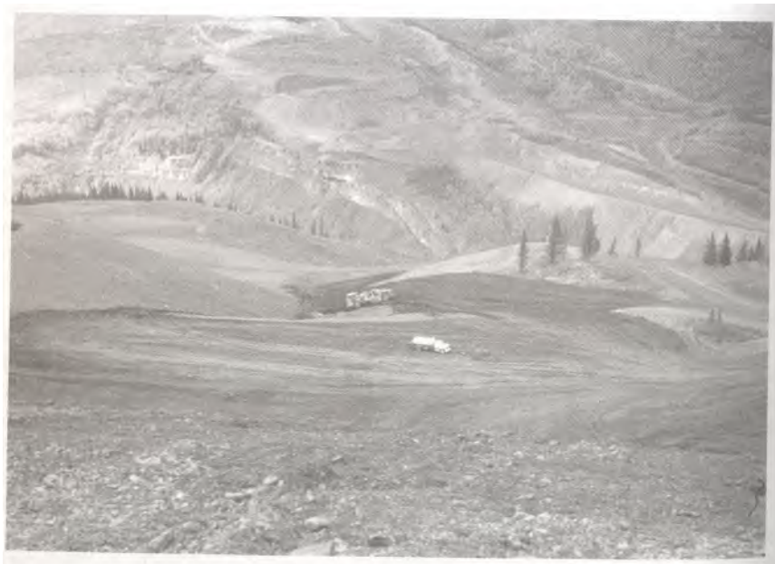
Fig. 21-6. Soil material previously salvaged and stockpiled is replaced following spoil grading.
