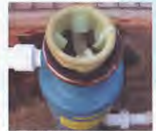
Water enters into a final metal filter that passes through a woven "sock." The weave of the sock determines the filtration level.
