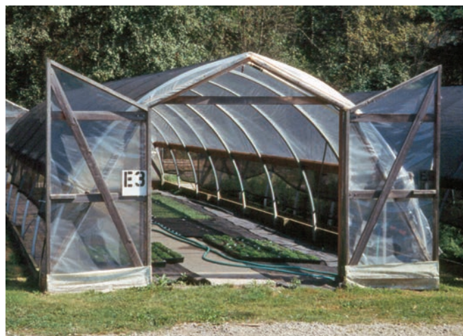
Figure 7.4.9 —Cloches and polyhouses are simple overwintering structures covered with white plastic (A) or Microfoam ® sheeting (B). The ends or sides are opened during warm and sunny winter weather for ventilation (C).
