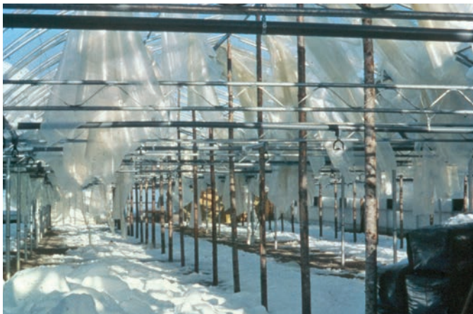
Figure 7.4.11 —Fully enclosed greenhouses are not good for overwintering, especially in climates with sunny winters (A and B). Snow removal is necessary in cold climates (C). Retractable roof greenhouses (D) are better for overwinter storage because they can be opened to allow heat to escape and snow to cover seedlings.
