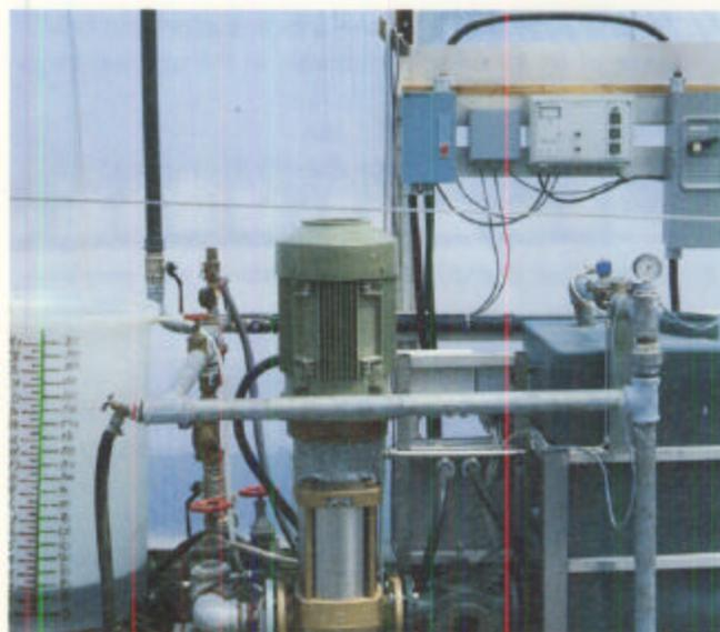
Figure 4.1.16—Injection of liquid fertilizers is an efficient fertilization method, but nutrient injectors should be designed to be compatible with the irrigation system.
