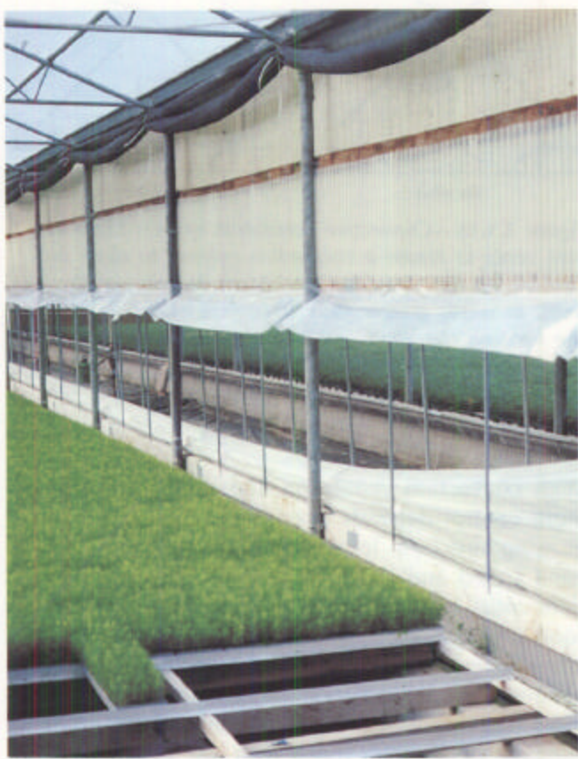
Figure 3.1.14 —Greenhouses with Poly-vent® sides can deflate the panels to generate good cross ventilation during hot weather. During the winter, the sides can be inflated to provide heat insulation.
