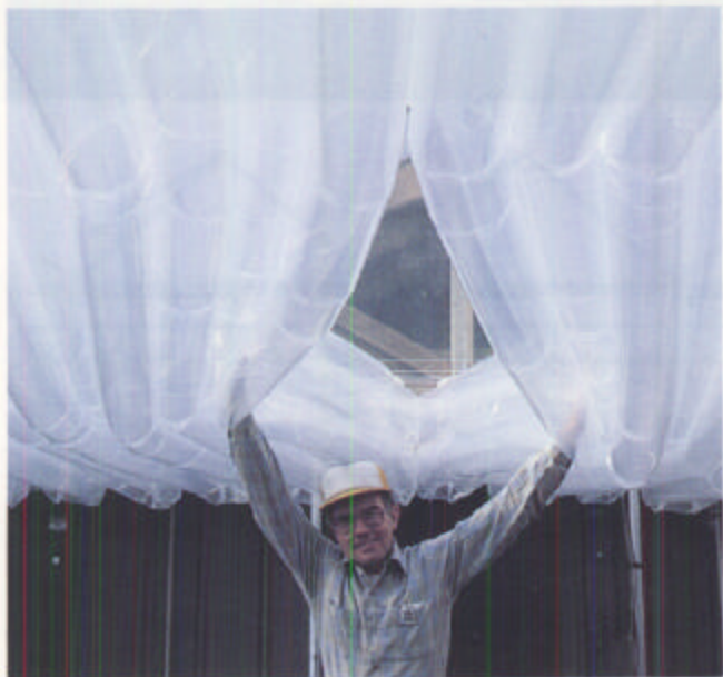
Figure 3.1.30 —Greenhouses can lose heat up to 10 times as fast as ordinary structures, and so insulation should be added along the north walls (A) and around the perimeter below bench height. Inflatable plastic ceilings can also be installed overhead (B).
