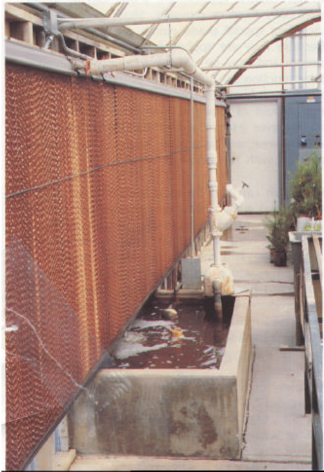
Figure 3.1.19 —A typical evaporative cooling system (A) consists of a specially designed wet pad on one end wall and exhaust fans on the other. A recirculating pump system (B) keeps the pad wet (C). The latent heat of evaporation lowers the temperature of the air coming through the pads and the cool air is drawn across the greenhouse.
