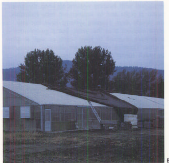
Figure 3.1.21—Synthetic shadecloth, traditionally used to cool greenhouses, is installed and left on throughout the summer months (A). When light intensity declines in the fall, shadecloth must be removed (B).
