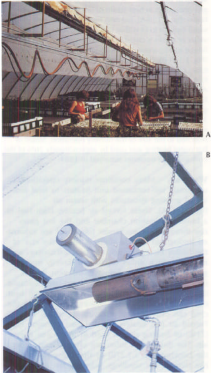
Figure 3.1.28—Overhead radiant heaters (A) warm objects (seedlings and workers) without raising the temperature of the surrounding air. Gas is burned in combustion chambers located along the heat pipe, which is equipped with metal shields to reflect the infrared radiation downward (B).
