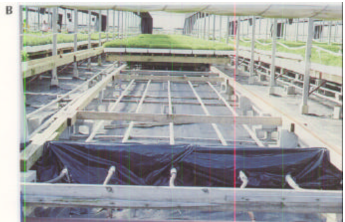
Figure 3.1.26 —Central heating systems use a large boiler (A), generally located in a separate building, to generate hot water or steam that is distributed through pipes to heat a number of surrounding growing structures (B).
