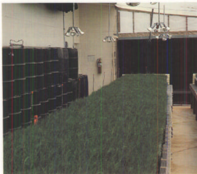
Figure 3.1.25 —Although many systems have been designed for greenhouses (A), few forest nurseries rely solely on solar heat. Container nursery managers can, however, modify their growing structures to capture solar energy and retard its loss at night. Black barrels filled with water are heated by the sun during the day and give off heat at night (B). (A, courtesy of D.H. Willits.)
