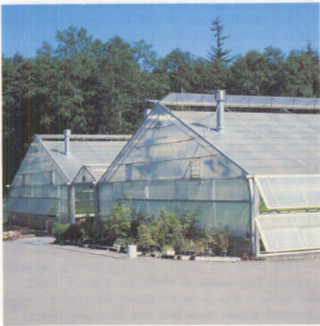
Figure 3.1.12 —The type of growing structure has a significant effect on the degree of temperature control that can be achieved and the cultural methods that can be used. A fully controlled environment (A) has heating, cooling, and forced air circulation capabilities. A semi-controlled environment, such as this shelterhouse (B), has forced air heating but also features roll-up sides that allow the grower to regulate temperature with cross ventilation. In recent years, container tree seedlings have been grown in outdoor "growing compounds" (C) that have no temperature control at all.
