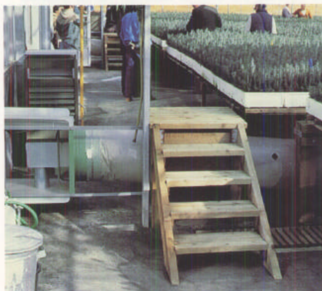
Figure 3.1.27 —Unit heaters are relatively small and are located in each growing structure (A), where they can be positioned to distribute heat directly to the seedling crop (B).
