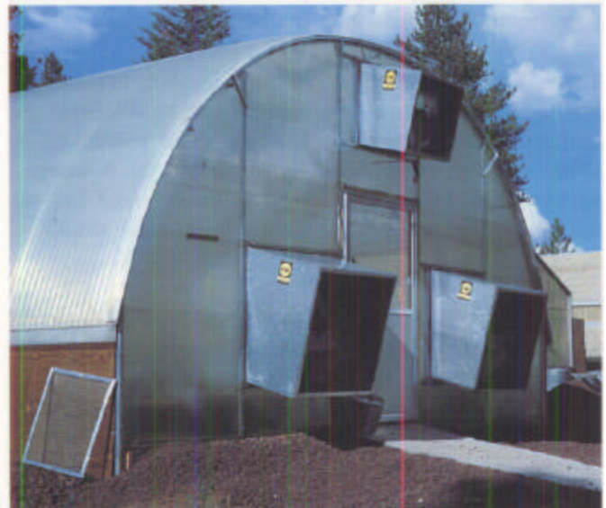
Figure 3.1.15 —A fan ventilation system greatly increases the air exchange rate and hence the cooling capacity of a greenhouse. A typical system consists of louvered vents on one end wall (A) that open automatically when the exhaust fans on the other end (B) are turned on.
