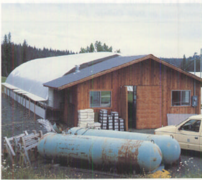
Figure 3.1.23 —Propane gas is a popular fuel for heating greenhouses in remote forest nurseries.
