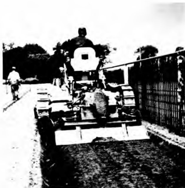
FIGURE 16.—A tractor-mounted bed shaper which forms and levels a seedbed in one operation. Bessey Nursery, Halsey, Nebr.
